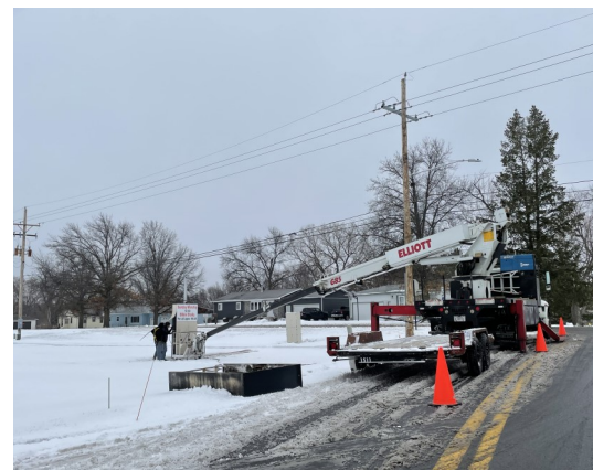
Mayhew Sign company digging footings for the new sign and pouring concrete to secure the steel posts.
