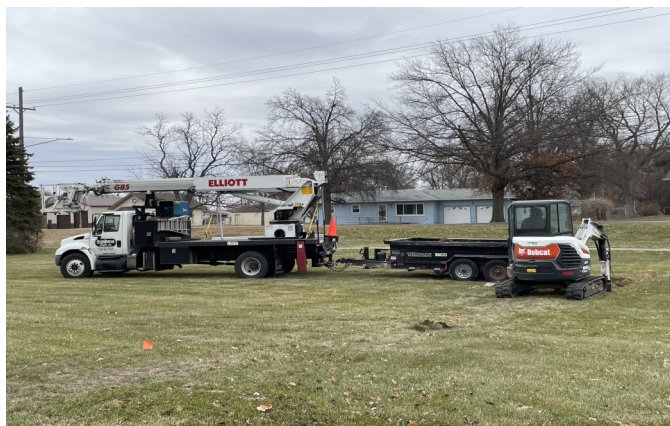
Mayhew Sign company digging footings for the new sign and pouring concrete to secure the steel posts.
