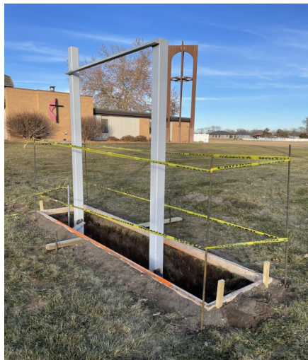
Mayhew Sign company digging footings for the new sign and pouring concrete to secure the steel posts.
